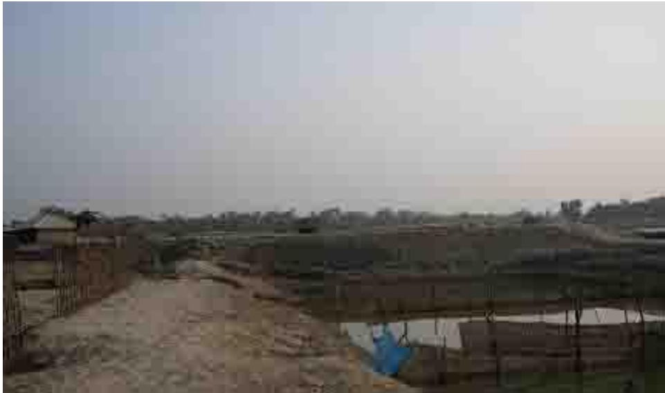
Figure-3: Embankment repair by CCEC
